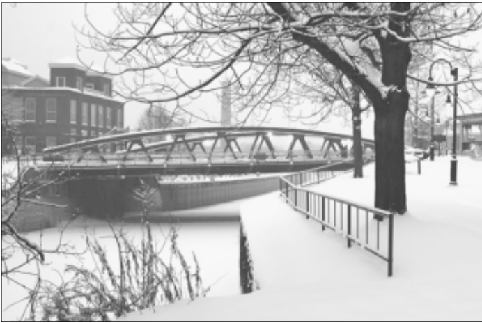
Fairport's historic lift bridge during a recent snowstorm. The bridge will be 100 years old this year! Photo by Keith Boas
